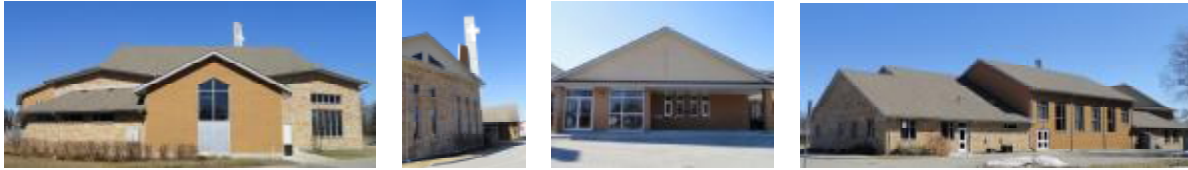
Sanctuary (S. & E. views) Main Entrance: Narthex & Offices CE Wing - Gym - Kitchen
